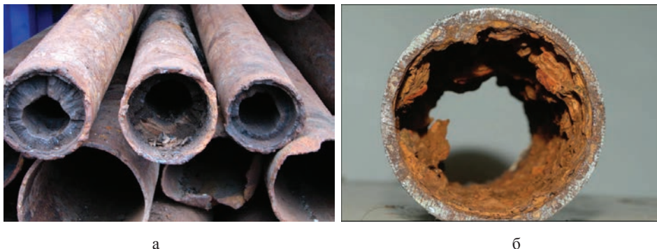
Fig. 1 (a, b) strings, exposed to corrosion and accumulation of salt deposits on their inner walls
